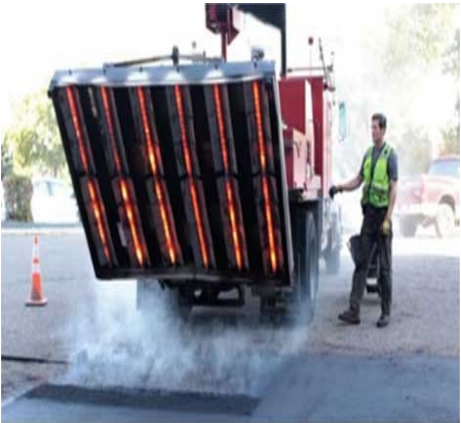
Infrared Patching Erickson Asphalt
