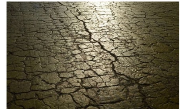
Oxidation breaks down and dries out the once flexible liquid asphalt that holds the aggregate together. This causes raveling and shrinking cracks which allow water to penetrate beneath the surface.
